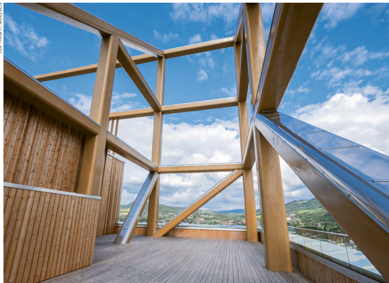
The 85.4 m and 18 storeys high Mjøstårnet is officially the world's tallest timber building.
